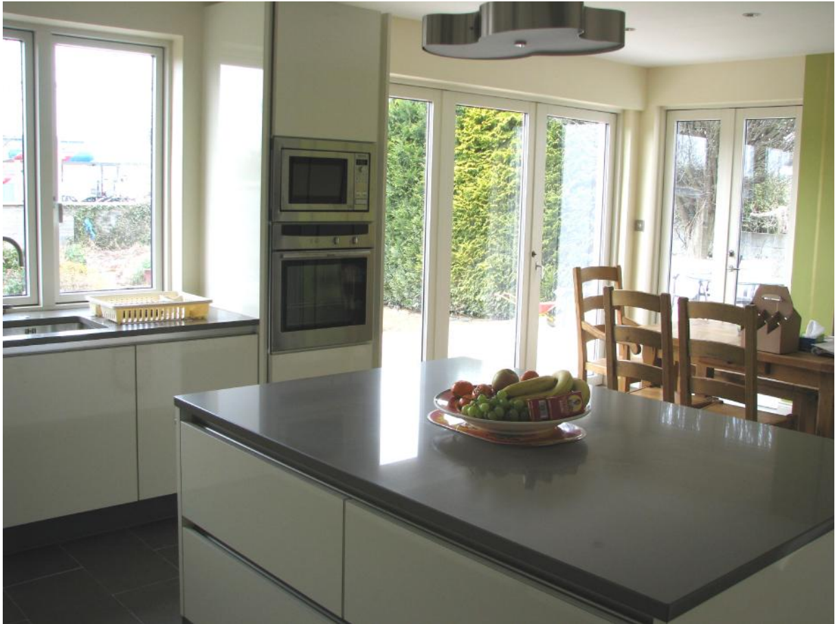
Dundrum, Kitchen design and refurbishment New windows + corner glass folding doors, new kitchen + new finishes. High gloss magnolia handleless finish with Silestone worktop
