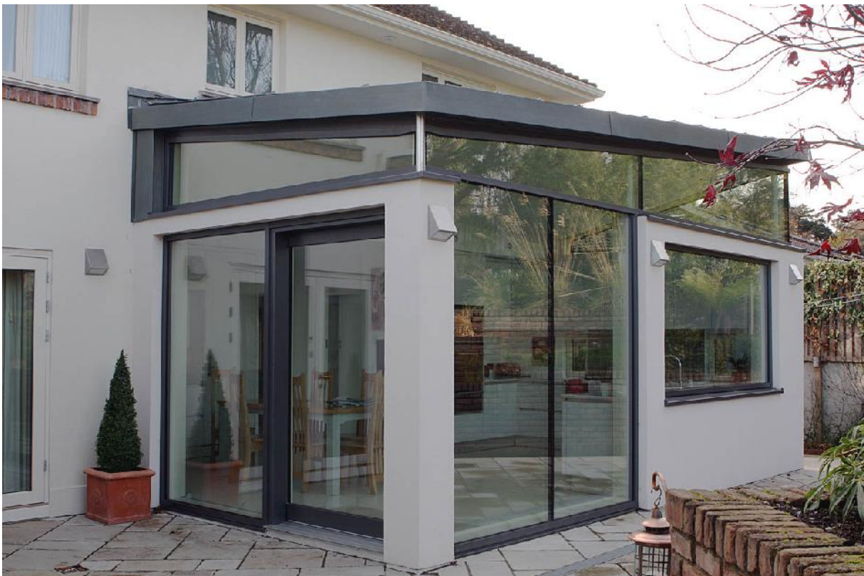
Use of post/beam window construction, with all-glass corners and butt-joint glass joins. All glass triple glazed. External insulated render system.
