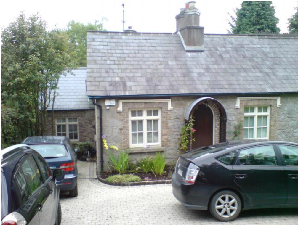
Enniskerry, Cottage, Extension, Renovation, Landscaping
