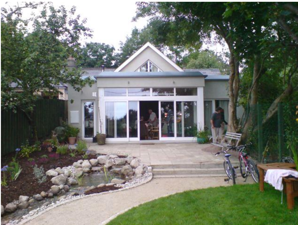
Enniskerry, Cottage, Extension, Renovation, Landscaping
