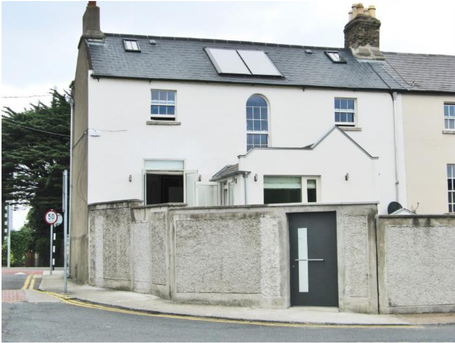
rear view. New access door, solar panels in roof, altered window openings to allow for more light
