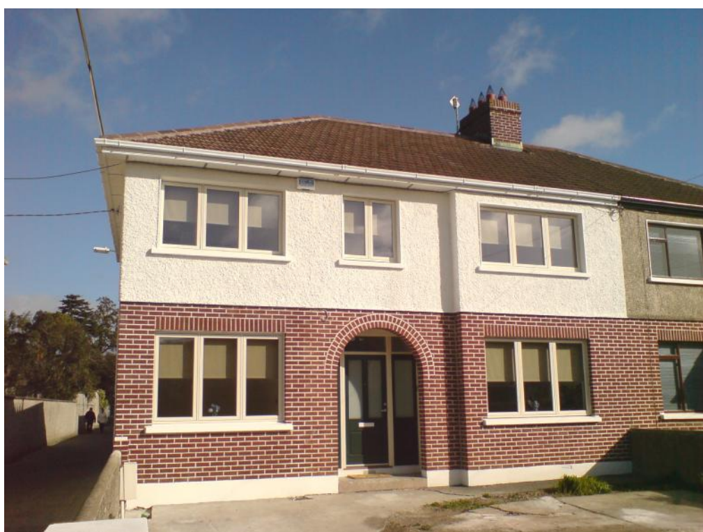
Mount Carmel Road, Goatstown 2 storey side extension to main house, to match existing materials
