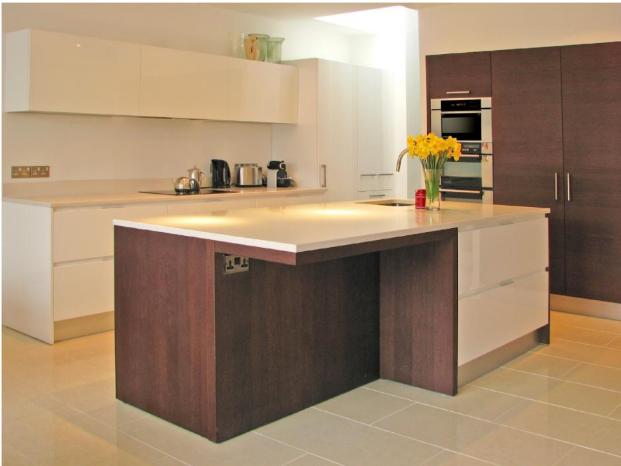
Kitchen project in Sandymount: Handle less high gloss polymer finish (postformed laminate rounded edge doors) in combination with Tecno oak veneer panels and doors. The tall units with veneered doors cover cylinder / boiler / hot-press behind. Silestone polished worktop to match the floor.
