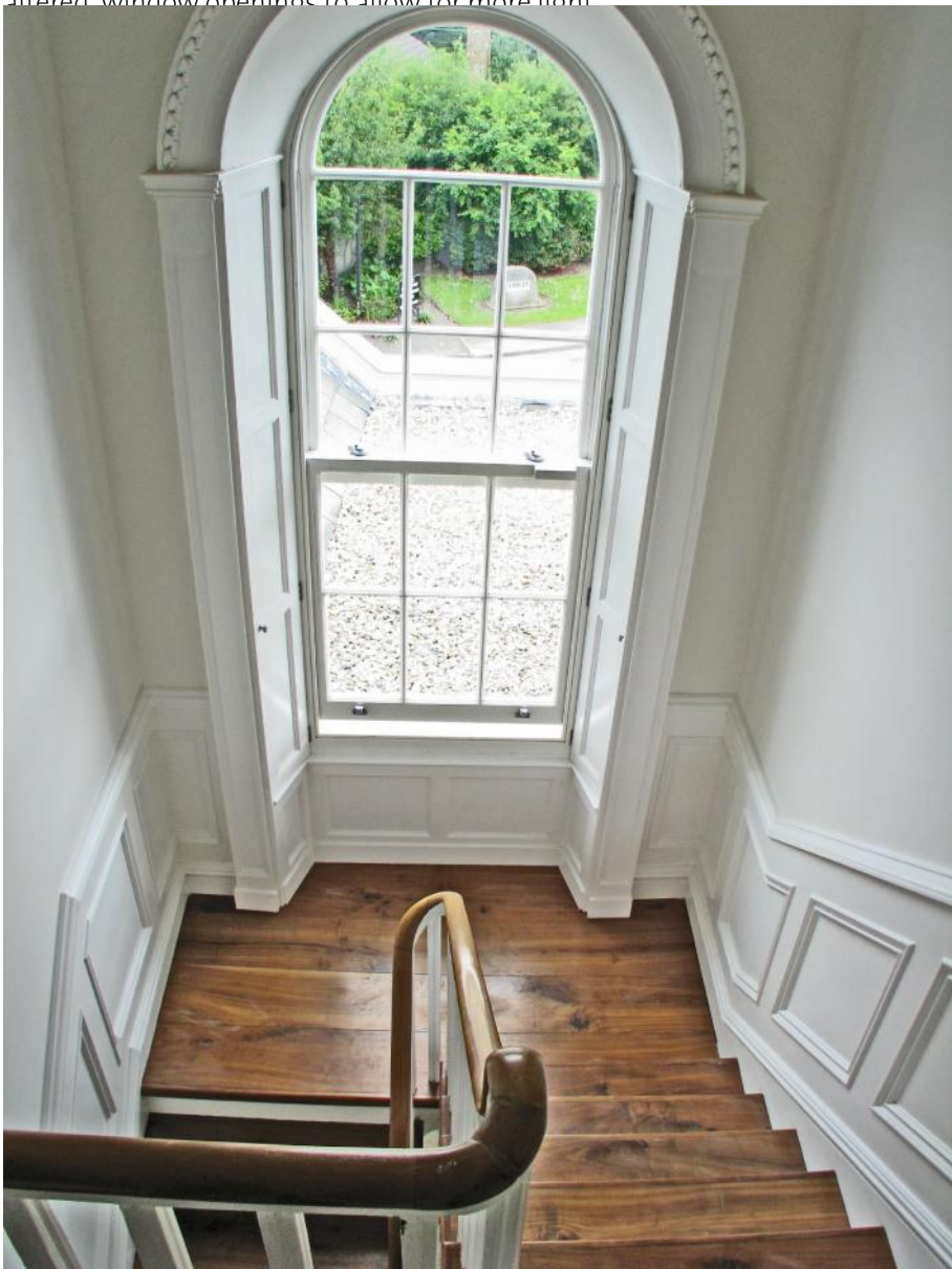
arched period window on half landing. New panelling to stairs
