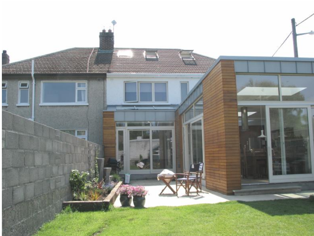
Mount Carmel Road, Goatstown Single storey rear extension with cedar cladding and zinc low pitch roof
