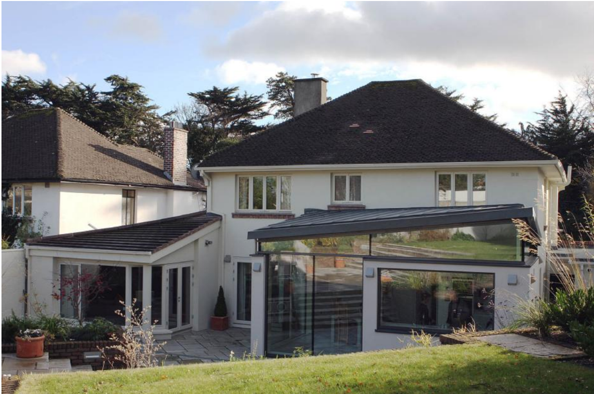
Rear extension to detached house in Blackrock. Roof is a double pitched zinc roof with a diagonal ridge. Designed to appear “floating” with glass wrap around.
