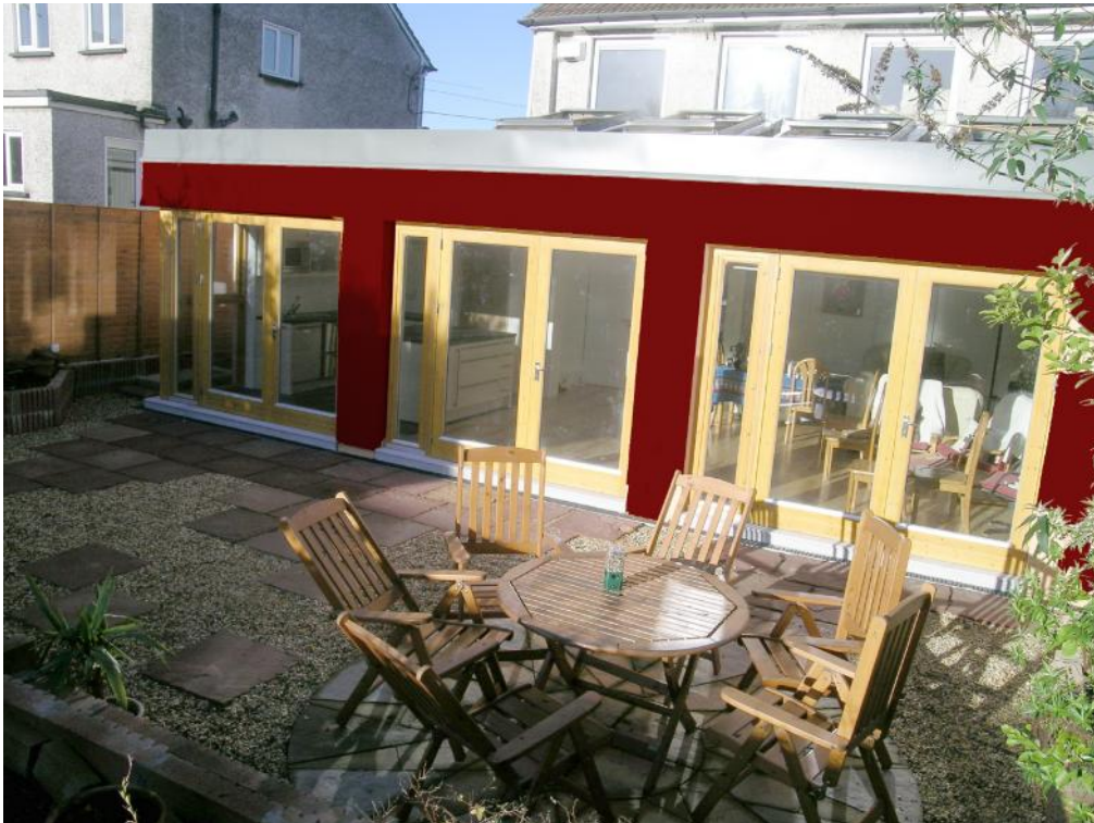
Dundrum, Rear extension with external insulated render system
